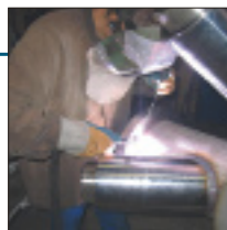
Experienced and qualified welders
