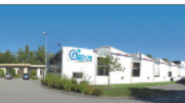
New production plant
